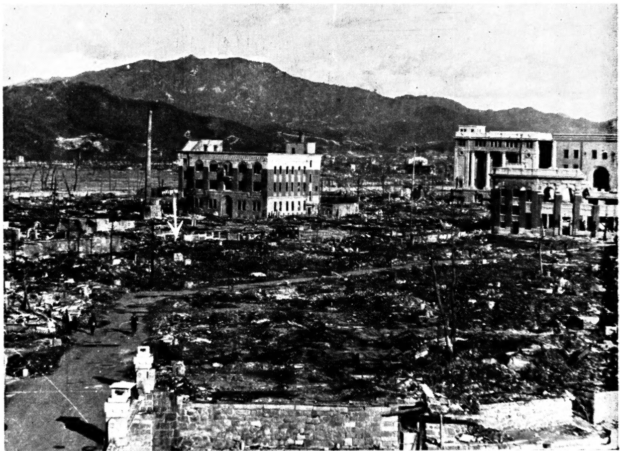
Photos Nos. 1 and 2. HIROSHIMA. General views looking across the centre of damage, the approximate position of which is marked with an arrow. It will be seen that some of the framed buildings quite near the centre remained standing. The tall building in Photo No. 1 is the same as that seen in Photo No. 7. The foreground illustrates the remnants of Japanese dwellings, razed to the ground. See paragraph 11.
